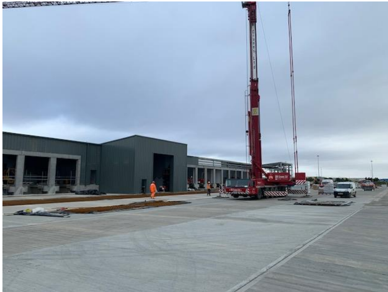
Construction of the new Border Control Post Facilities at Killingholme.
